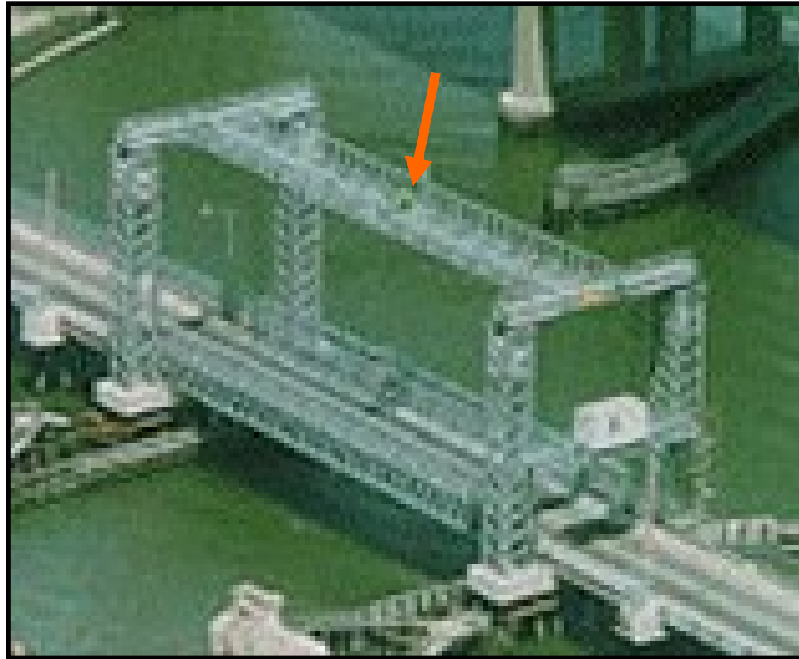
TOWER SPAN DRIVE
