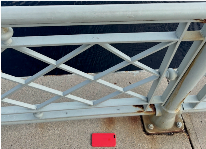
A smartphone placed on the sidewalk measures bridge vibrations on Boston University Bridge (Scott Snelling)
