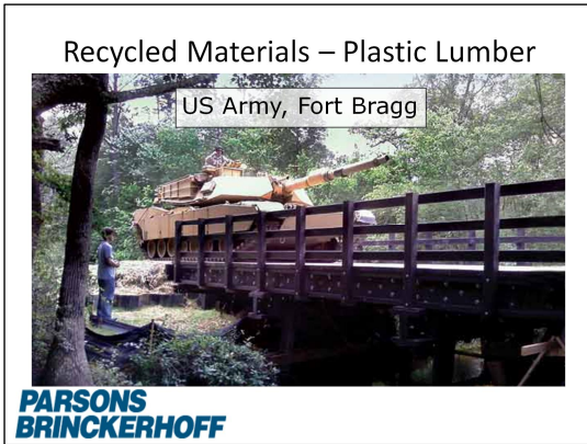
Bridge using structure of recycled plastic lumber was constructed at Fort Bragg in 2009. Designed by Parsons Brinckerhoff.
