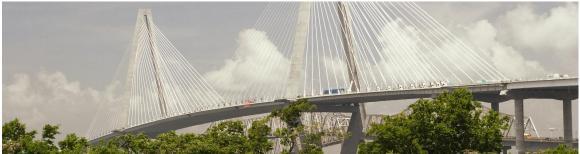
The Arthur Ravenel Jr. Bridge in Charleston, South Carolina is the longest cable stay bridge in North America; its construction was completed in 2005 using design-build project delivery.
