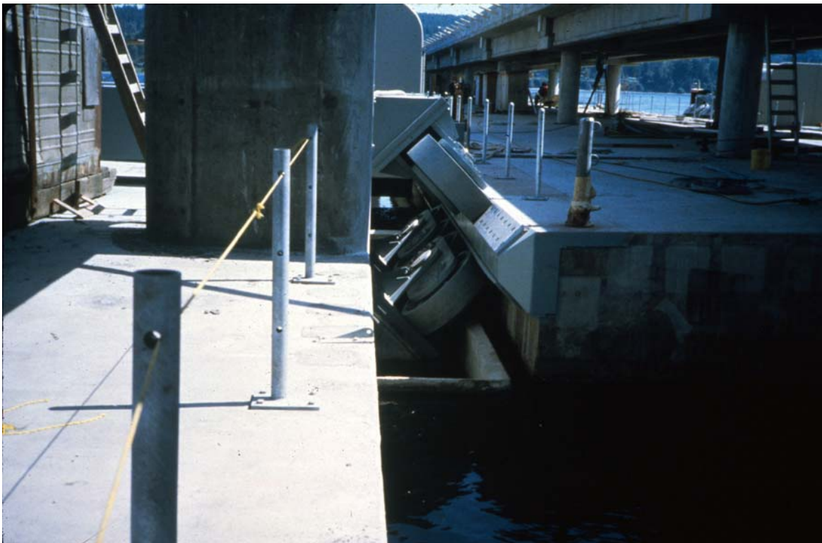
Figure 7 – 1982 Guide Rollers. Standing on Flanking Pontoon Looking Longitudinally
