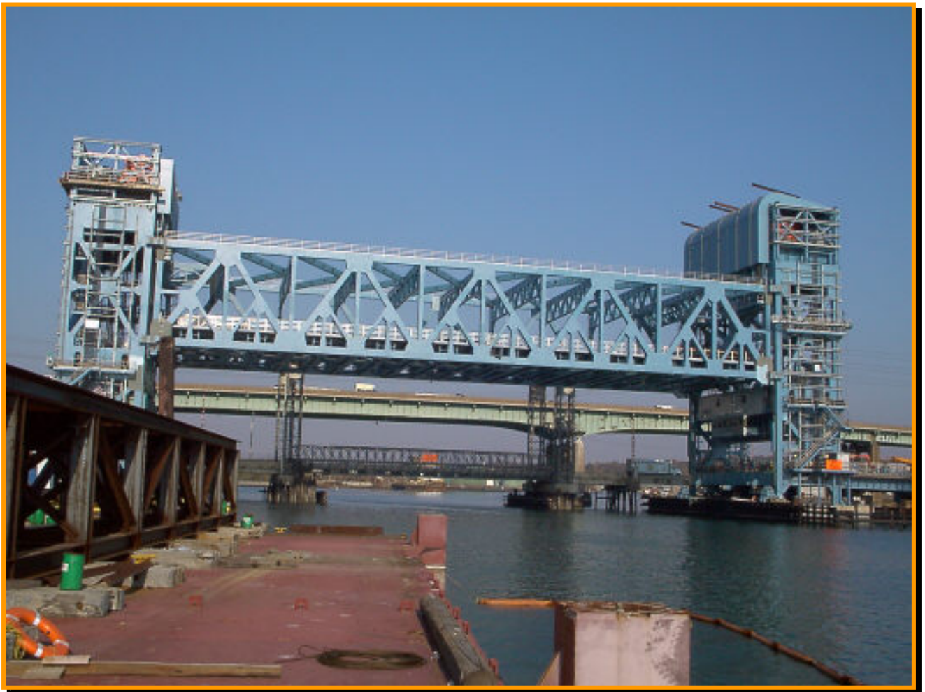
FIGURE 2.2 – Tomlinson Bridge: A Tower Drive Type Vertical Lift Bridge
